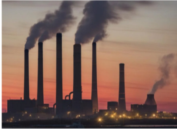
Mystic Natural Gas Generating Station
